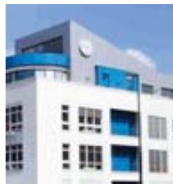
The DECHEMA building in Frankfurt am Main
